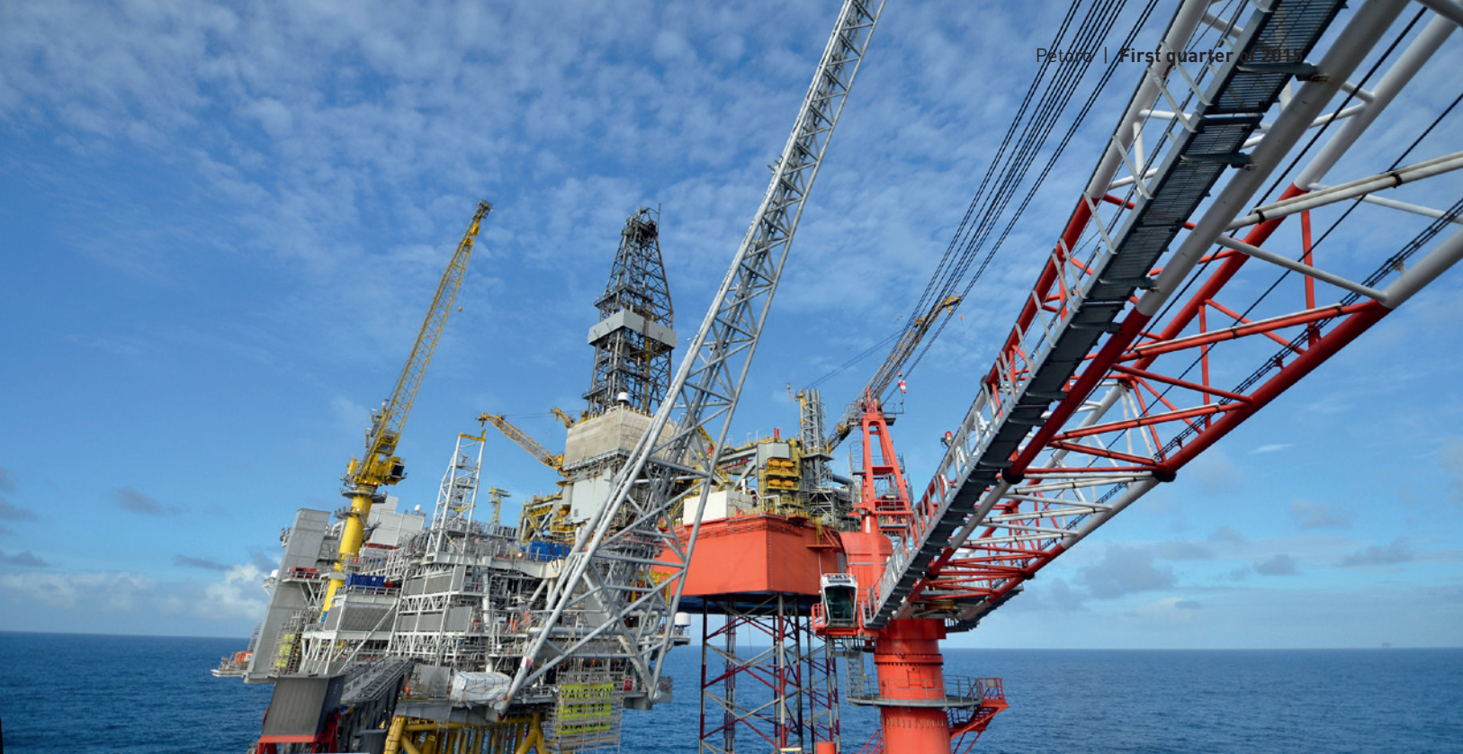
The Valemon field began production on 3 January 2015. Petoro is a partner with 30 per cent. Photo: Harald Pettersen/Statoil
